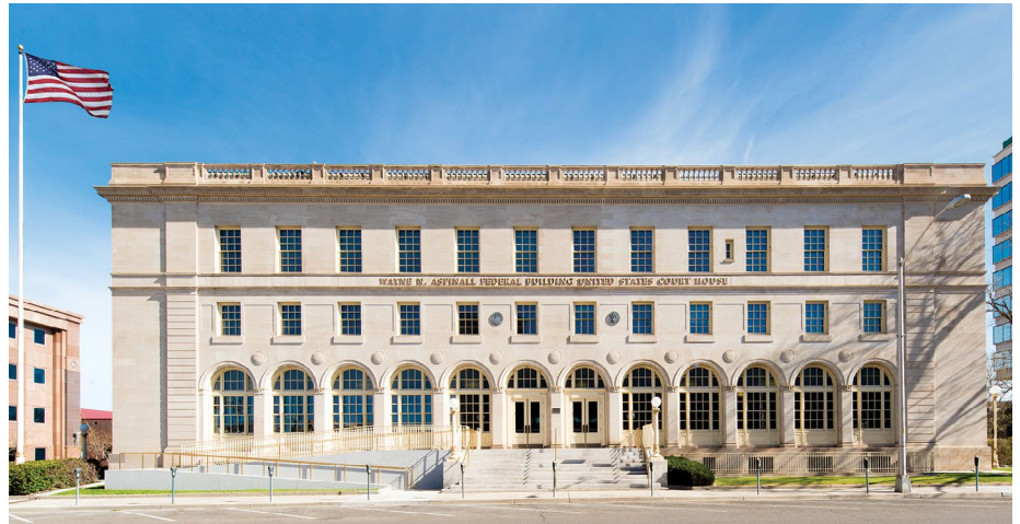
Figure 7: The Wayne Aspinall Federal Building and U.S. Courthouse, Grand Junction, Colorado. Photo by Kevin G. Reeves, Courtesy of DLR Group|Westlake Reed Leskosky.
