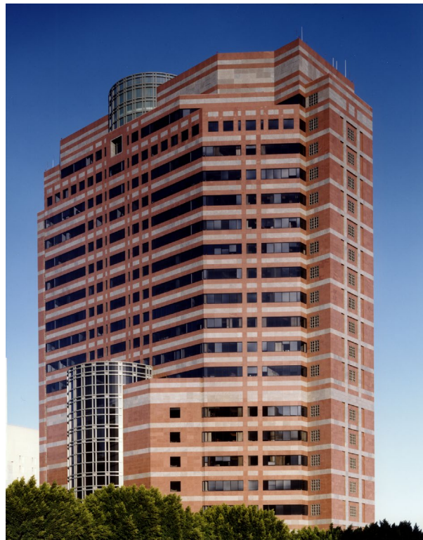
Figure 12: The Edward Roybal Federal Building, Los Angeles, California
